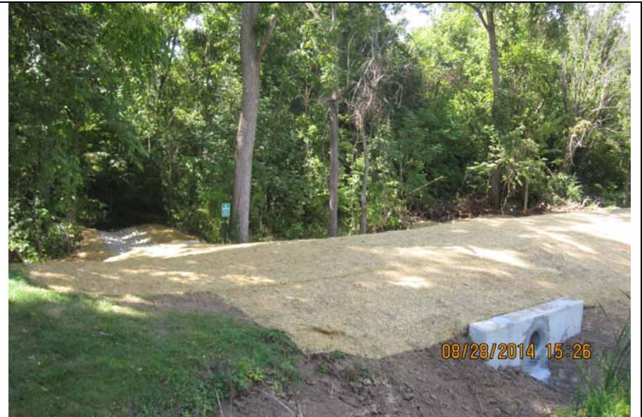
Photo #6: Installed new concrete culvert and headwalls.
